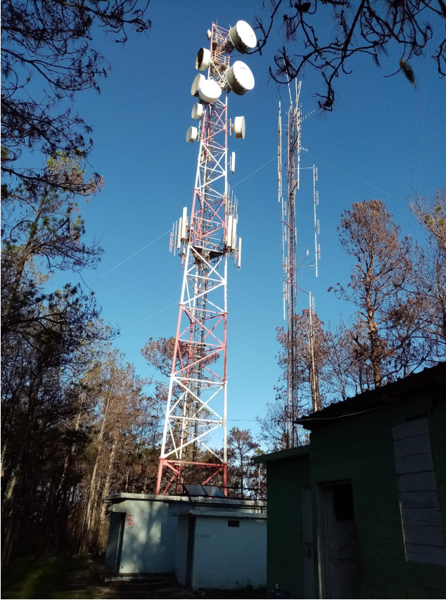
Photo 1: Altice communication tower in the background
