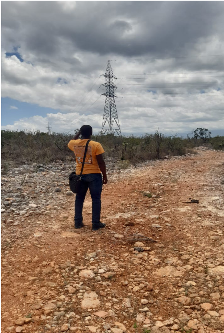
Photo 12: Measuring height of power line tower with height meter
