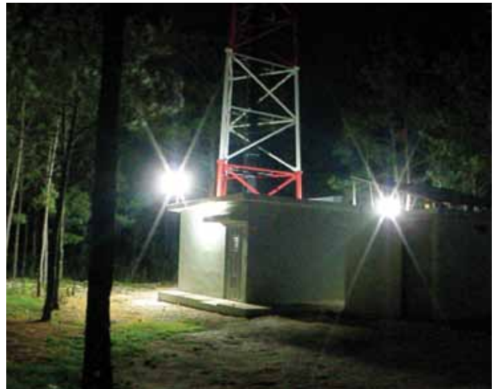
This brightly-lit cell phone tower is within 30 m from the cliff where petrels breed at Loma del Toro, Dominican Republic. The lights are likely to attract petrels to this tower, and two nearby guyed towers, creating a fatal threat to breeding petrels at this site. Photo: Goetz, 2009
