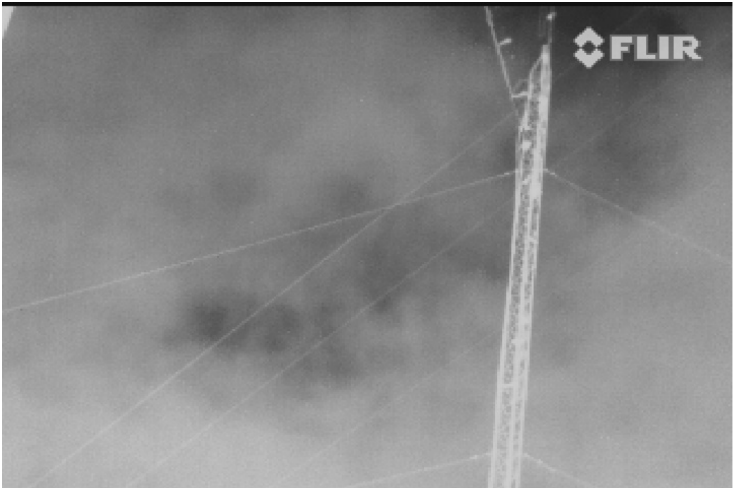
Figure 1: Photo of the high tower with guy wires taken with the thermal camera
